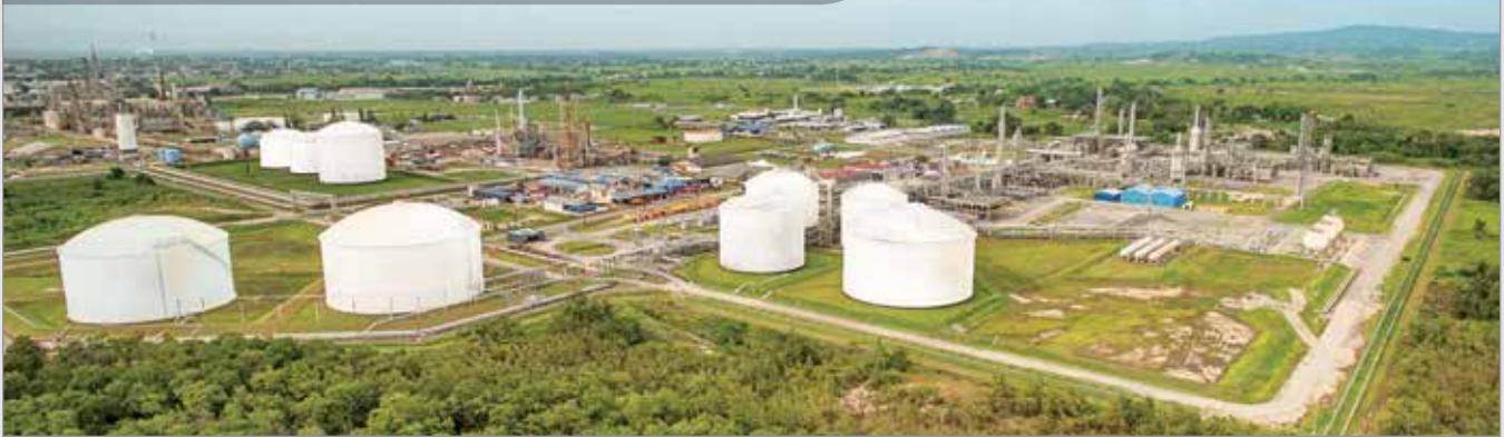
PPGPL's Facility at Point Lisas
