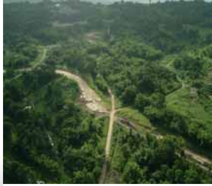
ROWs being cleared at Union Estate
