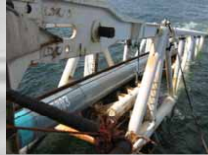
Pipe being Lowered into the Water
