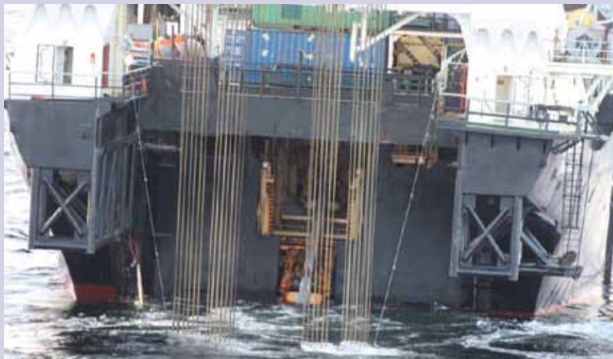
Pipelaying in the marine environment.
