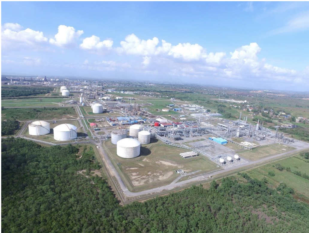
Aerial View of the Point Lisas Industrial Estate
