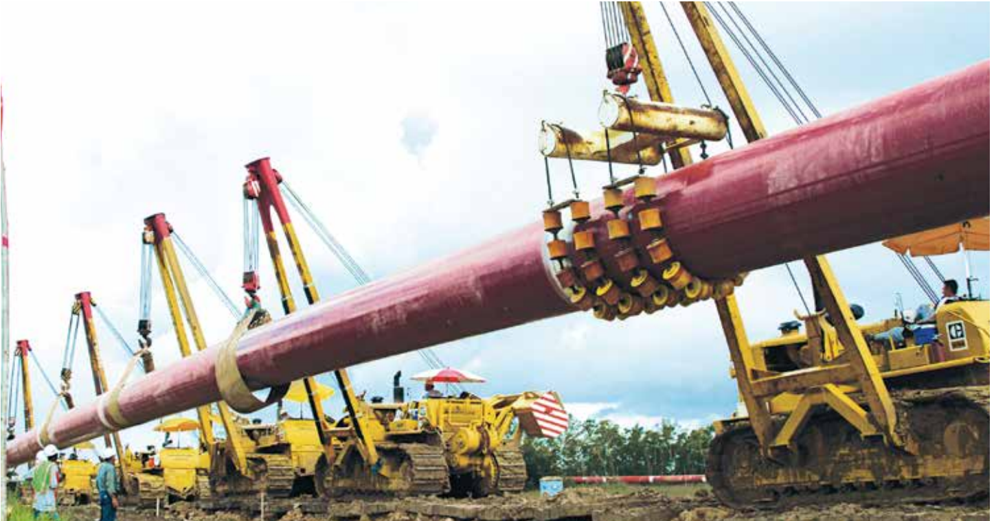
56-inch Cross Island Pipeline under construction
