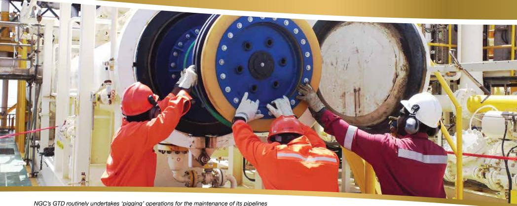
NGC's GTD routinely undertakes 'pigging' operations for the maintenance of its pipelines
