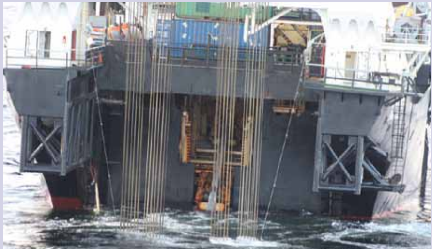
Pipelaying in the marine environment.
