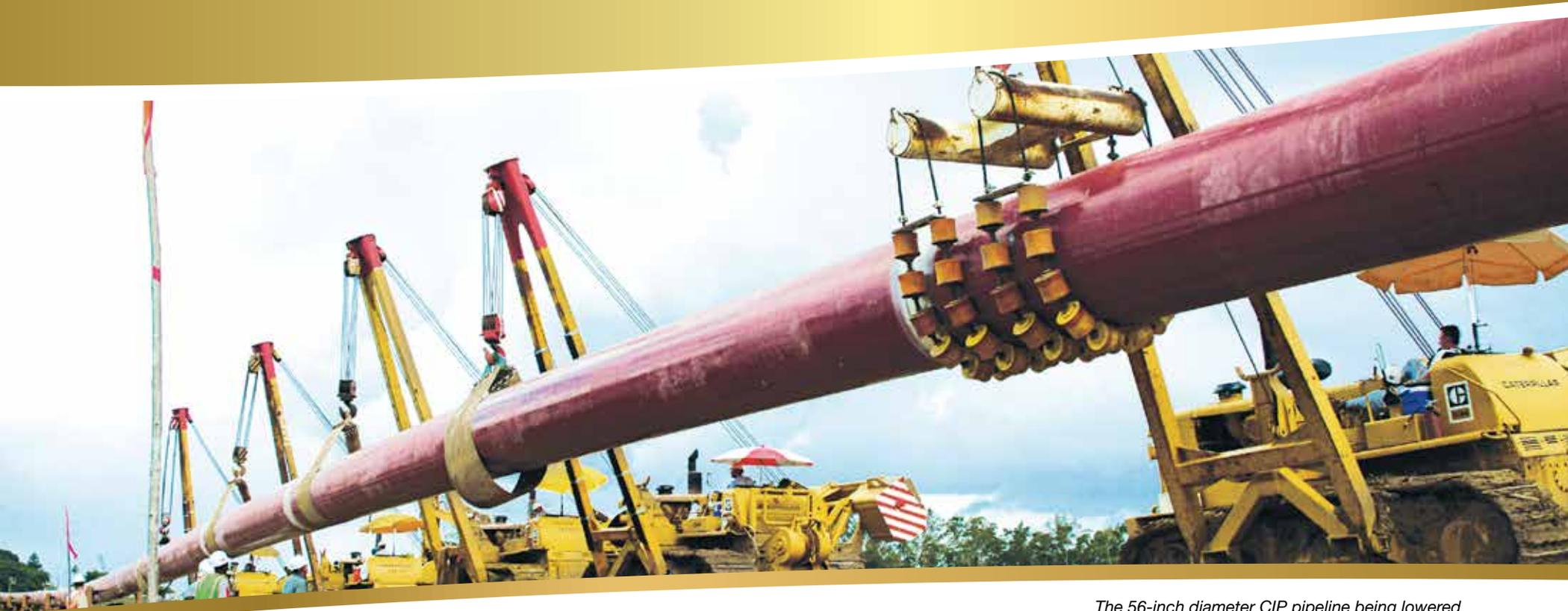
*The 56-inch diameter CIP pipeline being lowered*
