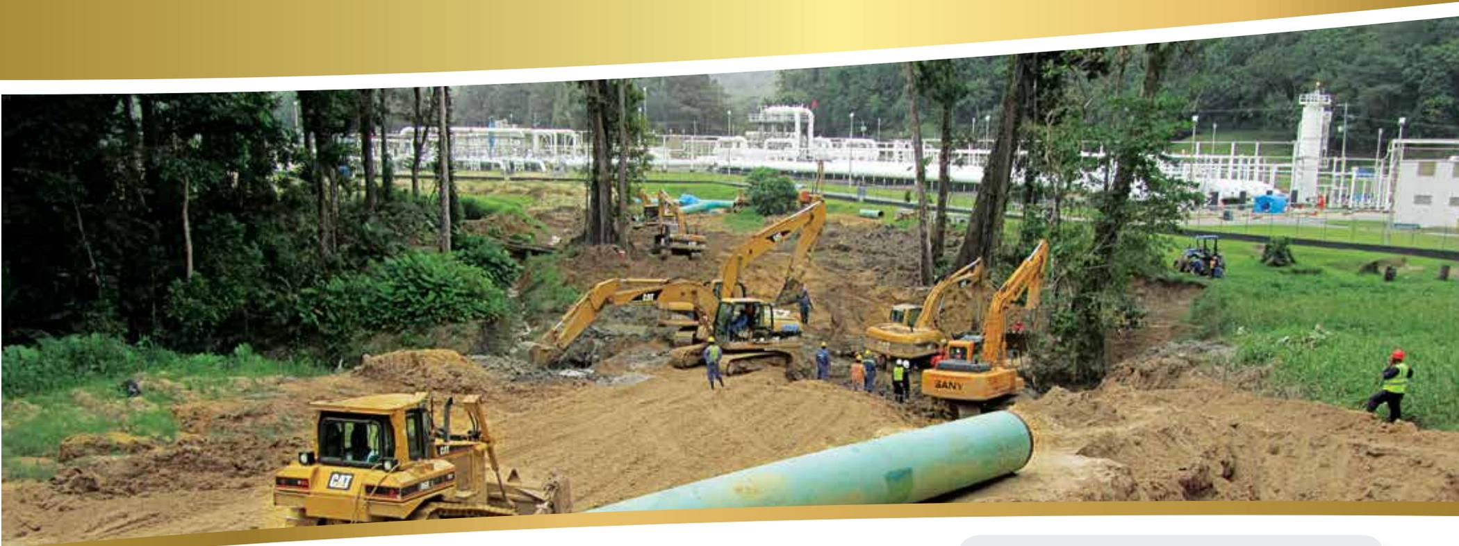
*Onshore pipeline construction in progress for the North-Eastern Offshore (NEO) Pipeline Project*
