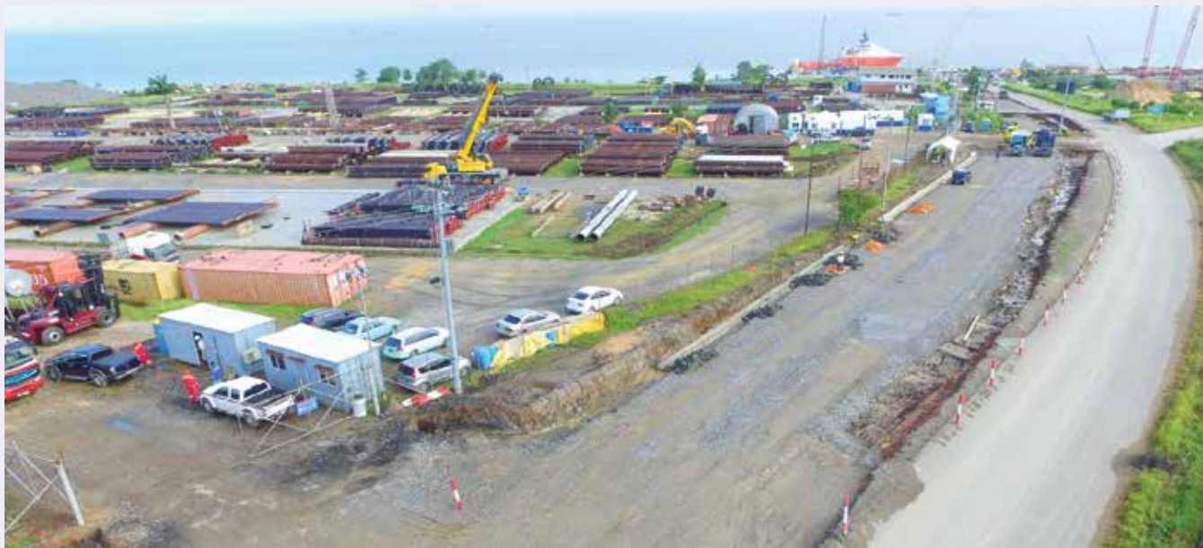
Reconstruction of the LABIDCO Corridor and Pipeline ROW Project: The project entails widening and realignment of the existing roadway
