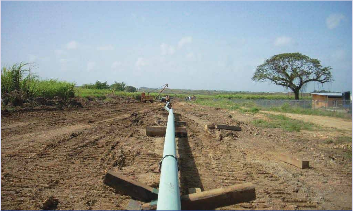
Pipelaying – Liquid Fuels pipelines
