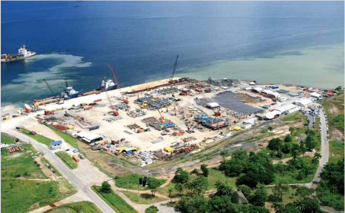
Fabrication Yard – Brighton Port, La Brea.
