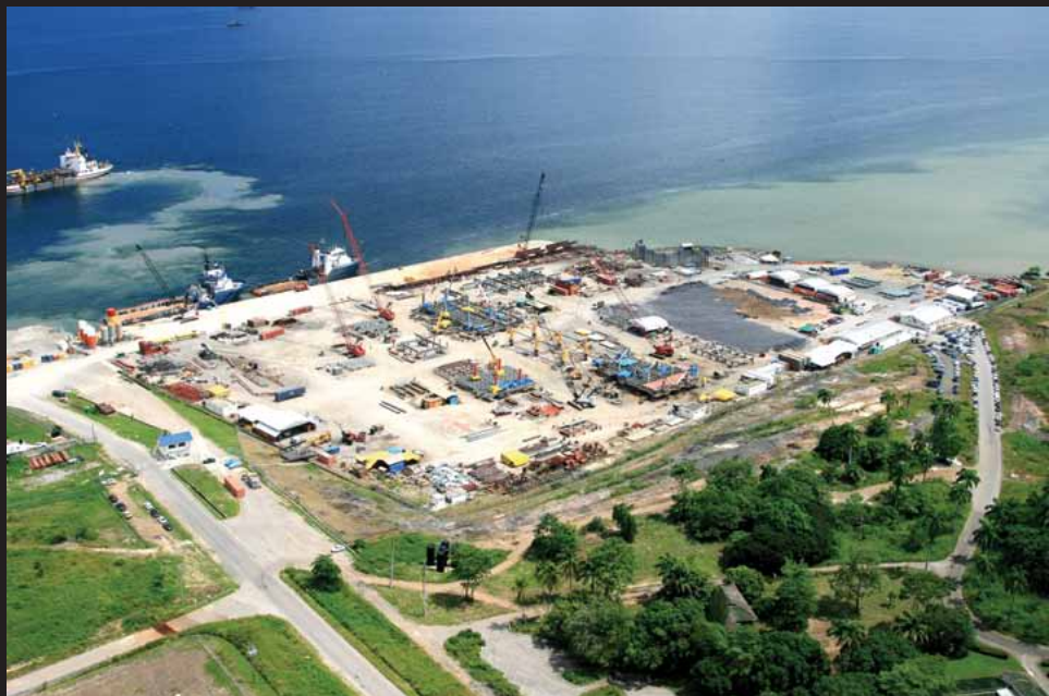
Brighton Port with Fabrication Yard in foreground.
