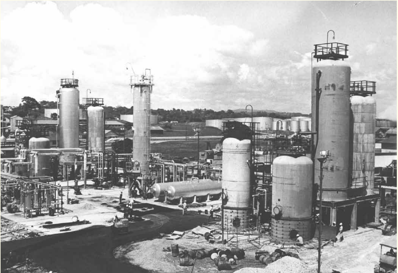
Early refinery at Pointe-à-Pierre.
