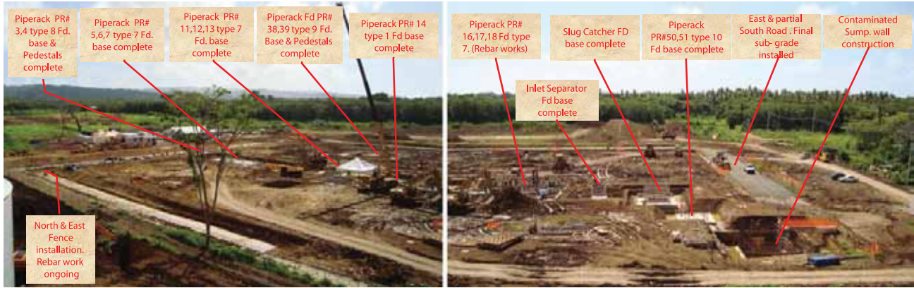
Gas Receiving Facility – Tobago Pipeline Project.
