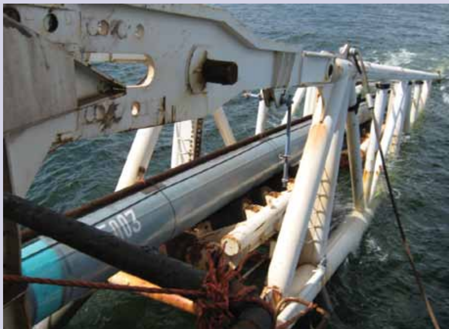
Marine pipelaying activities – Tobago Pipeline
