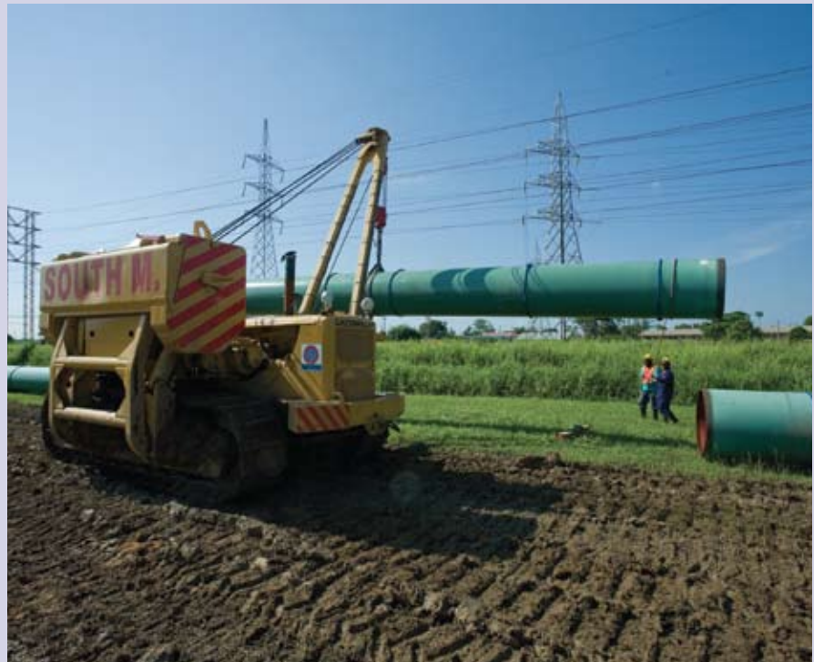
Pipelayering – hoop to ring main
