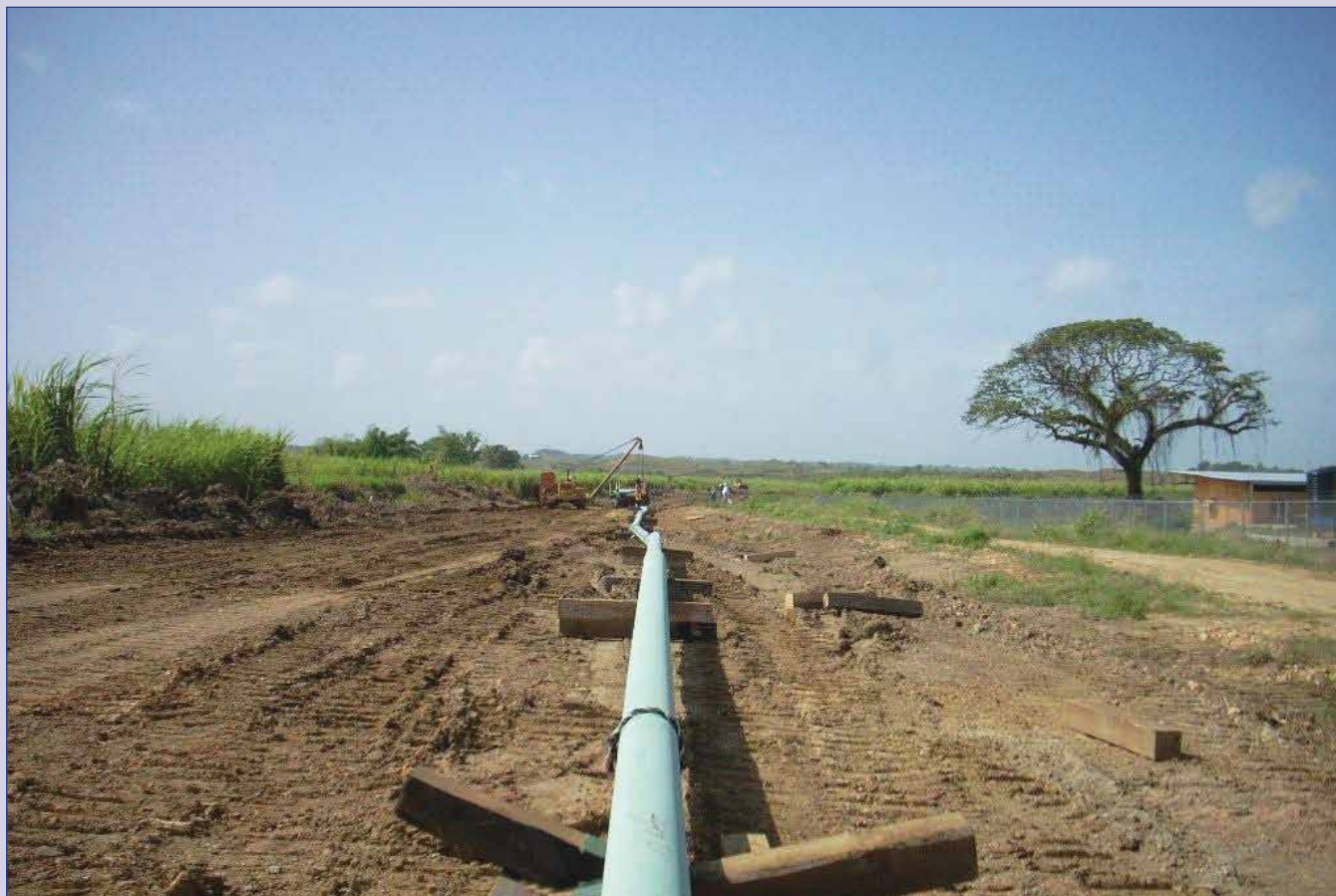
Pipelaying – Liquid Fuels Pipelines
