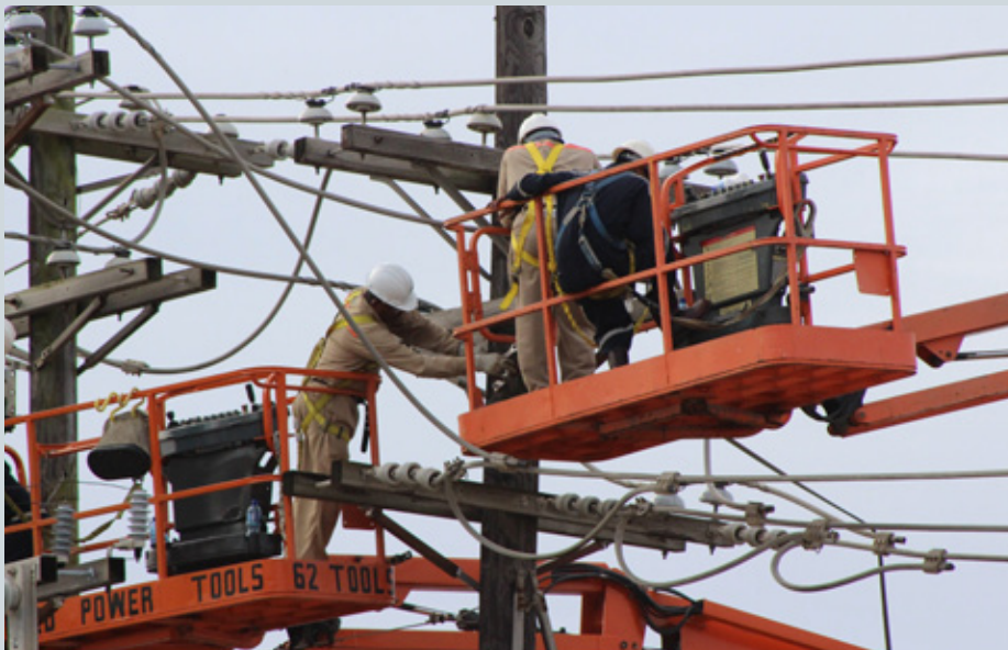
TTEC is executing maintenance works on PPGPL's 12KV Overhead Lines.
